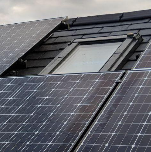
Thermostatically controlled roof light with rain sensor, connected to a tilt and turn cellar door for automated, rapid, passive cooling potential
