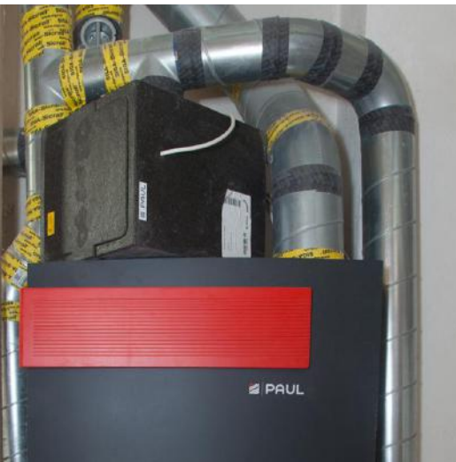
Paul Novus 300 heat recovery ventilation system - 93-94% heat recovery with a specific fan power of just 0.24 Wh/m 3
