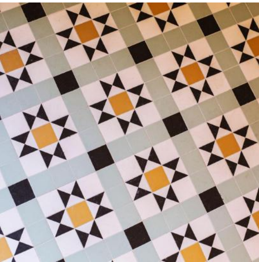
Breathable construction details throughout including lime grout and adhesive tiled floors
