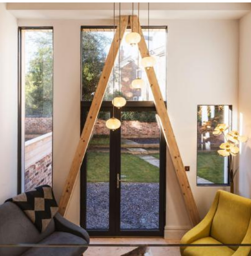
Structural timber V & A's for lateral stability in place of steel tie to drive down embodied carbon and reduce thermal bridging
