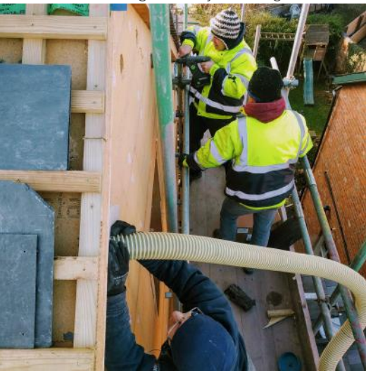
Blown cellulose insulation made from recycled newsprint salt treated for fungicide and fire offered very fast and flexible solution with enhancement of both U-Value and airtightness. Great for complex spaces.
