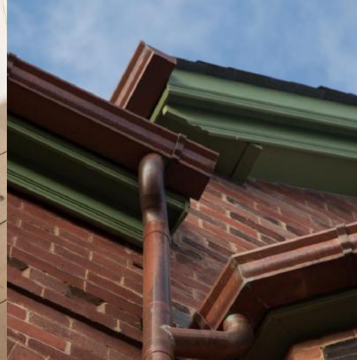
The copper guttering and downpipes are expected to last over 120 years!
