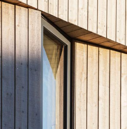
Articulated cladding is “pre-fossilised”, to resist rot and UV degradation for over 30 years maintenance free
