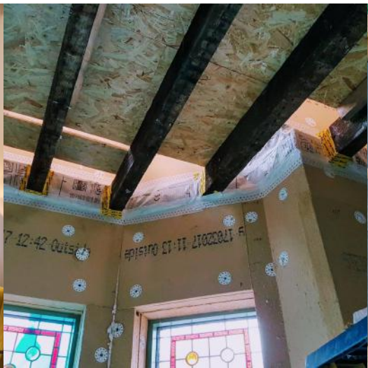
IWI system developed to retain the original bay proportions and window apertures of the victorian facade, high enough performance to achieve PH and retain full breathability avoiding petrochemical insulants
