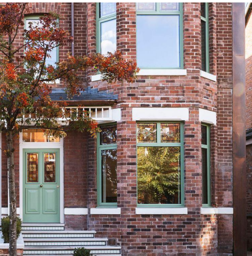
Insulated sidewall disguised by heritage sensitive, subtle copper coping that blends into the traditional brickwork.
