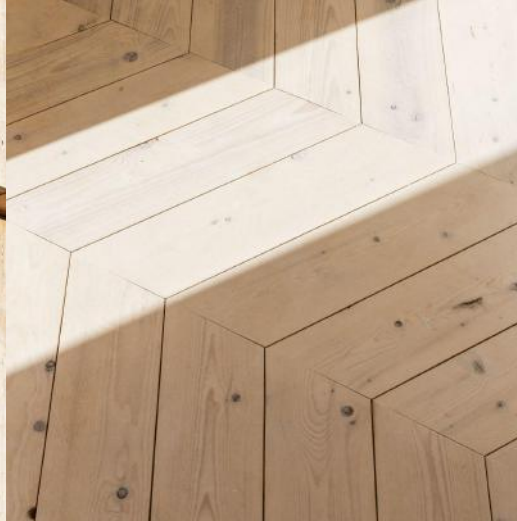
No extension to footprint and reuse of over 200 tonnes of brick the entire existing roof, stairwell and floor structures throughout with repurposed floor boards or in an effort to reduce embodied carbon and reduce landfill.
