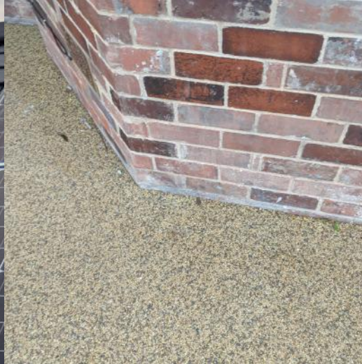
Sustainable Urban Drainage (SUDS) featuring recycled tyres and recycled stone aggregate for driveway and building surround greatly reducing potential water ingress to the cellar and provide mild flood resistance for the building
