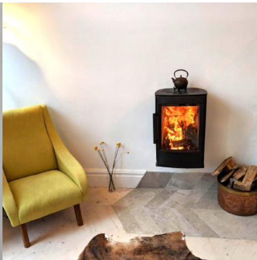
5kW DiBT accredited Log Burning Stove for backup (heat input not included in PHPP calculations).
