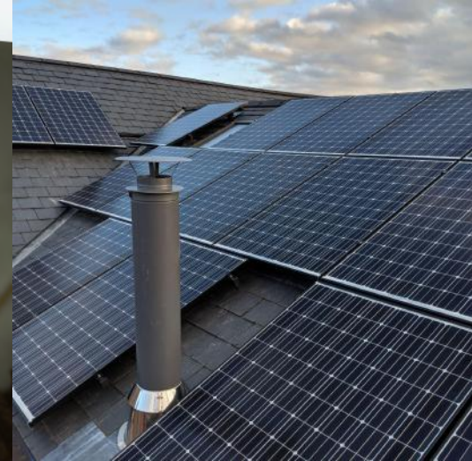
36 x 330-Watt Panasonic HIT modules over two systems. Tigo voltage optimiser to efficiently manage any shading effects and optimise even Northerly aspect panels. Wiring design optimised for later addition of on-site energy storage or EV charging.
