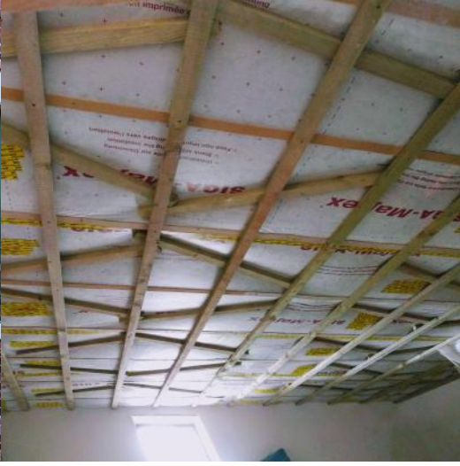
Hidden in the roof is another world first use of Siga's Majrex intelligent building membrane adopting cactus inspired biomimicry to keep the building fabric dry and airtight.
